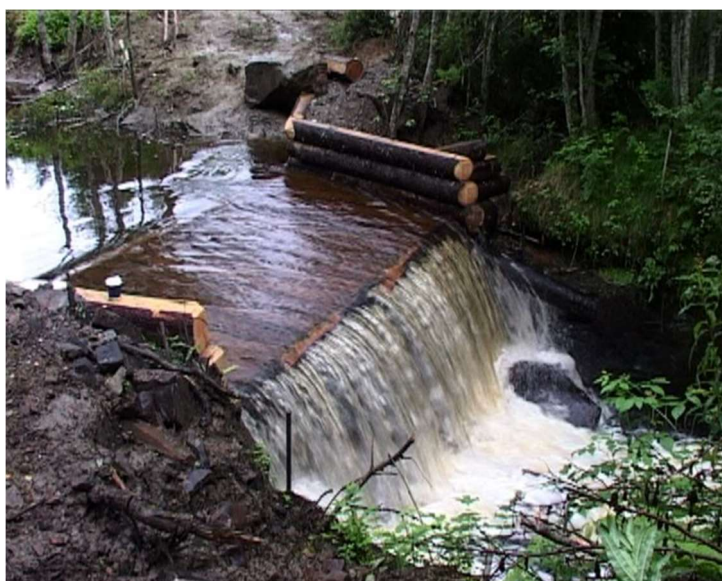
Fig. 2 Temporary barrier in a tributary of the River Ognå
