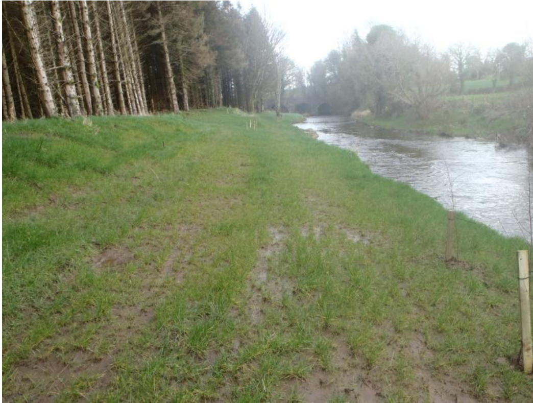
Berm-lowering to increase storage during flood events
