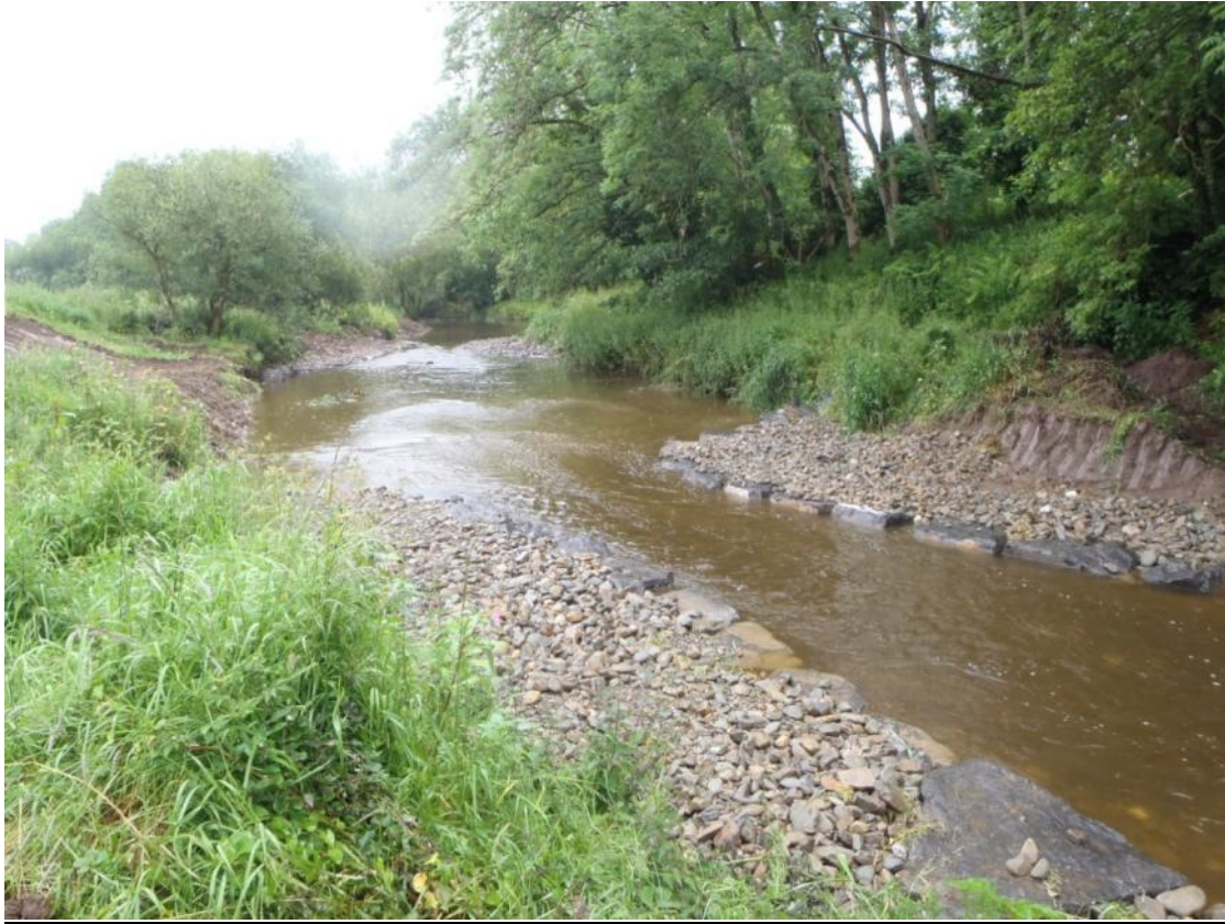
Low level D-groynes to increase low flow diversity
