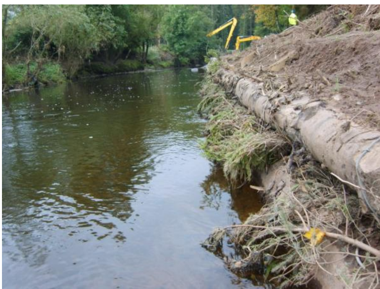
Fallen trees used as bank protection
