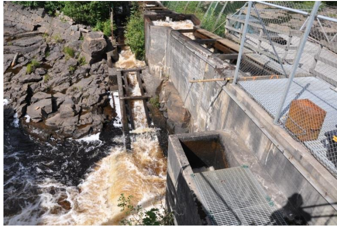
The Denil fish ladder built in 1946 in the River Ätran. Photo Hans Schibli.
