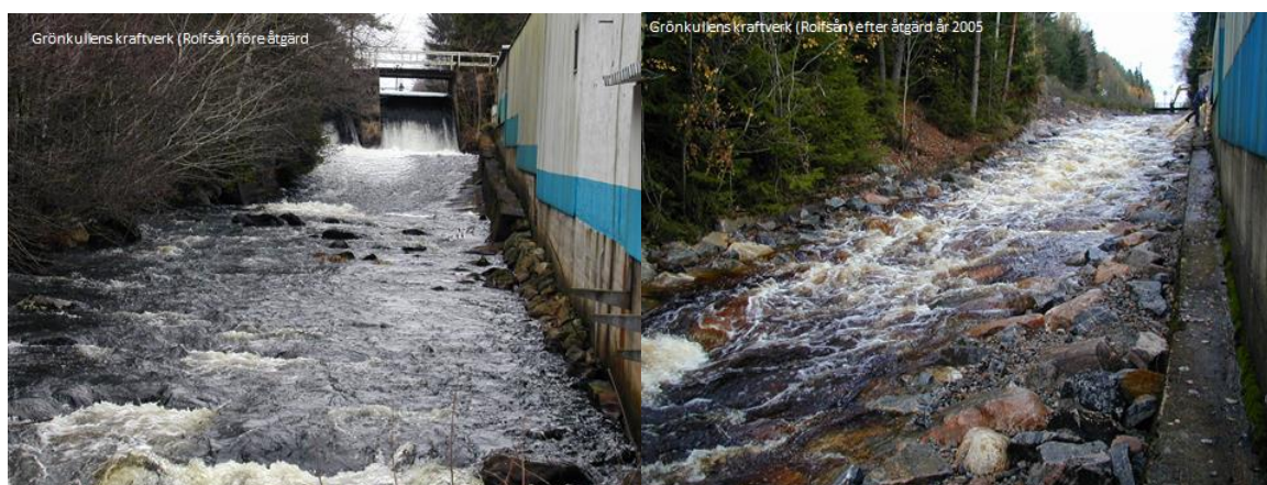
Before and after removal of a dam at a hydropower plant in the Atlantic salmon river Roflsån. The dam was replaced with a rocky ramp. Photo by Andreas Bäckstrand
