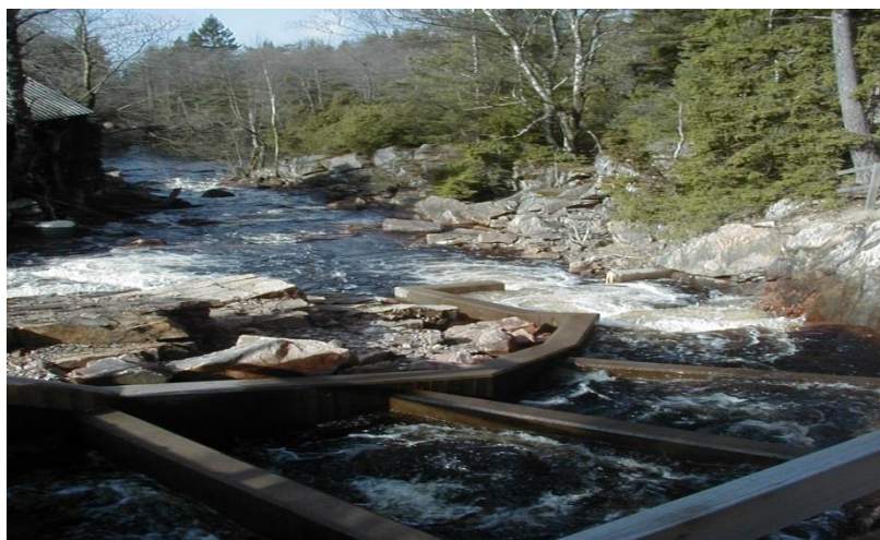
Pool and weir fishway in the Atlantic salmon River Nissan. Photo by Hans Schibllii
