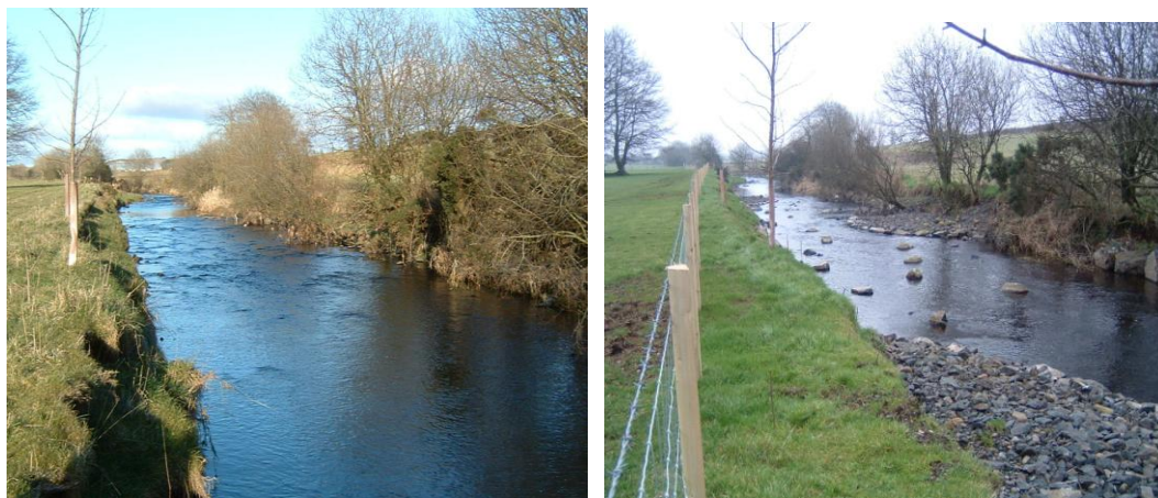
Figure 11. LHS Section of the River Main prior to enhancement work, this site was characterised by a lack of quality nursery habitat with limited stream bed cover, inadequate depth at summer flow levels and extensive bank erosion on the right hand bank. RHS Same section of the River Main after enhancement works. Flow deflectors, random boulders and fencing had been utilised to improve local salmonid nursery habitat
