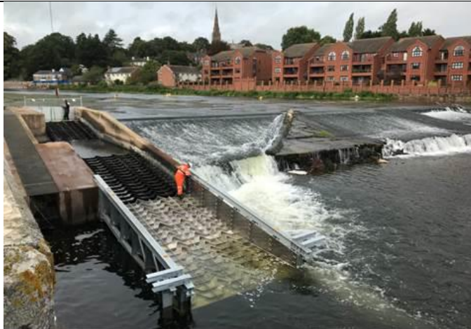
Trews Weir larinier fish pass on the River Exe
