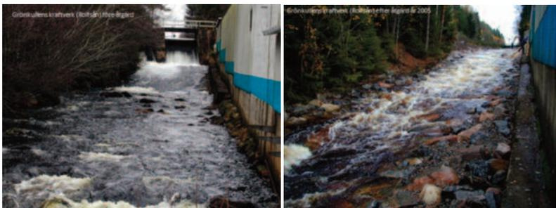
*Before and after removal of a dam at a hydropower plant in the Atlantic salmon river Roflsån. The dam was replaced with a rocky ramp. Photo by Andreas Bäckstrand*
