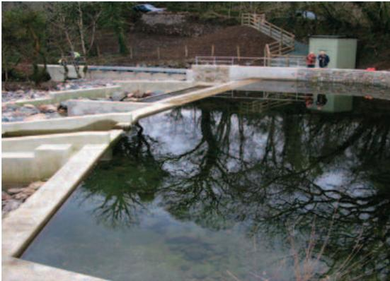
*Hill Bridge hydropower intake on the River Tavy in South West England - protected river flows, fish screening and improved fish passage saves hundreds of smolts every year.*
