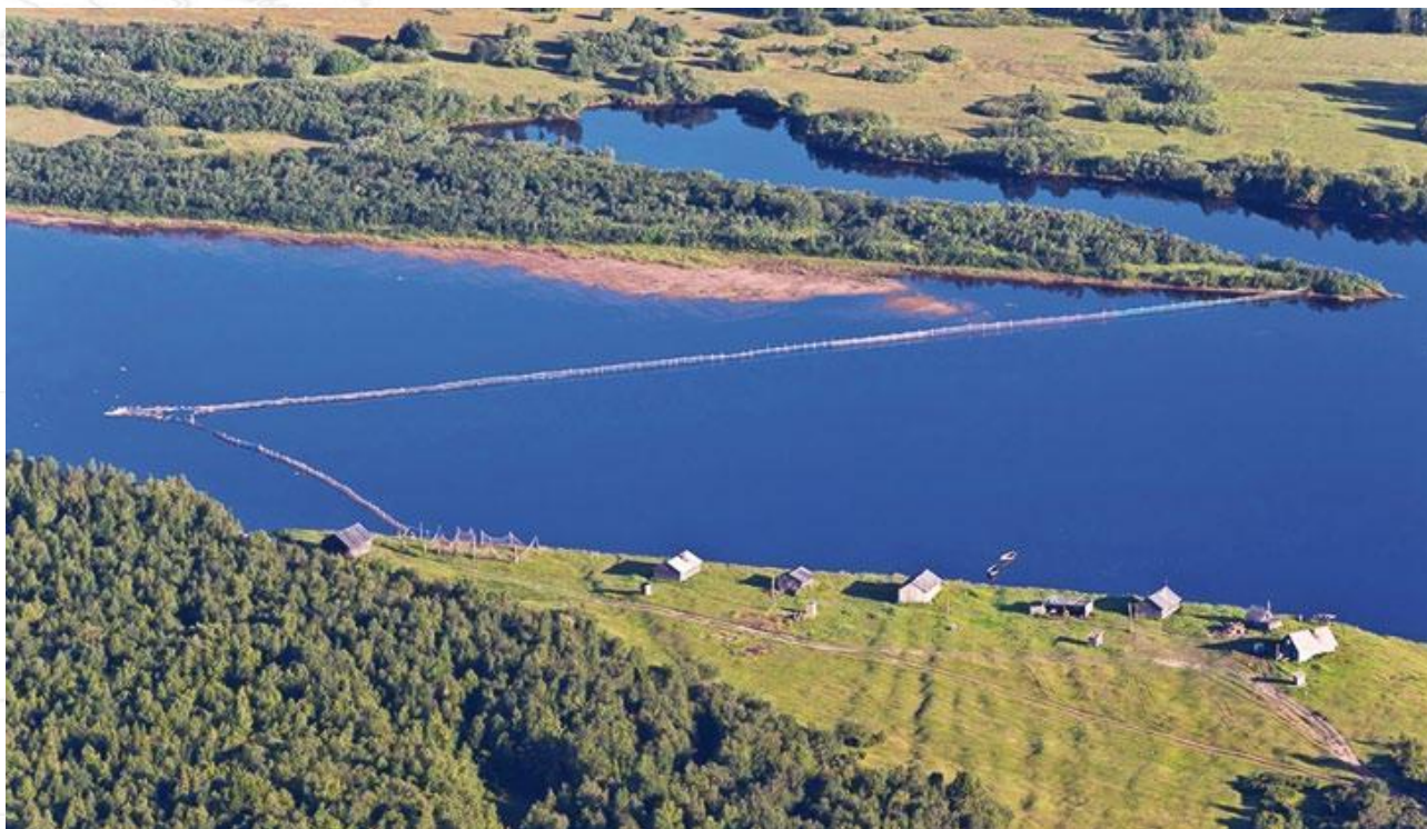
The barrier fence in the Varzuga River
