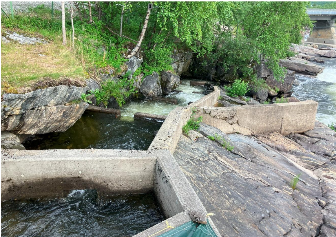
Figure 3. A fish ladder at Neidenelva leads up to the fish trap at the top. Credit: NASCO Secretariat.
