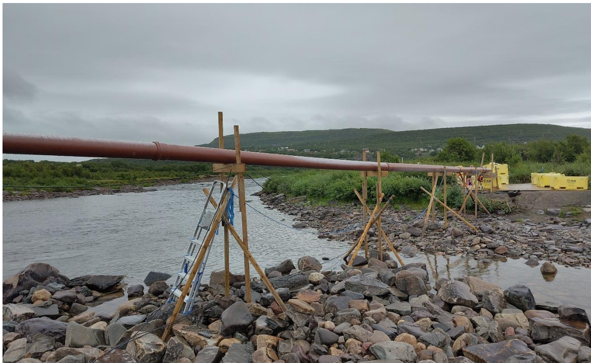
Figure 15. Fish transport system to move pink salmon from trap to fish boxes on the Vestre Jakobselva. Credit: NASCO Secretariat.
