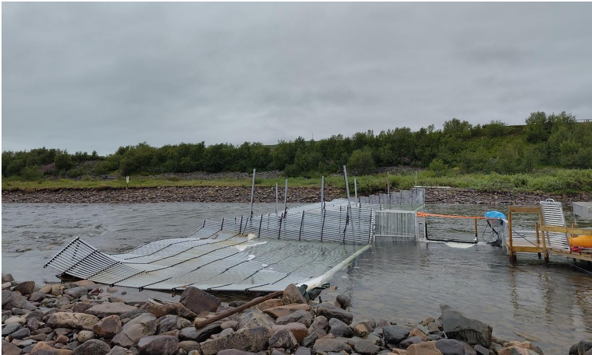
Figure 12. Floating fence and fish trap on the Vestre Jakobselva, with artificial intelligence prototype to automatically sort pink salmon from Atlantic salmon. Credit: NASCO Secretariat.
